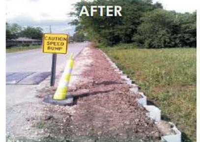
Due to the extreme slope of the land, this road in Lafourche Parish in Louisiana was cracking and sliding down the slope, causing unsafe conditions and resulting in ongoing repair expenses. The problem was corrected using Tidewall TW75 in 3 meter long sheets, with approximately 2/3 meter of exposed height. This brought the shoulder of the road closer to the elevation of the road itself, relieving the stress on the asphalt and allowing permanent repairs to be made.
