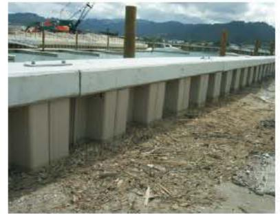
Tidewall sheets were used to construct a secure, permanent wall around a new high-end marina in Tauranga, New Zealand. Tidewall was chosen for its combination of aesthetics, corrosion resistance, and low cost. Precast concrete sections were placed atop the wall, and the final result is a beautiful wall that will last for decades.
