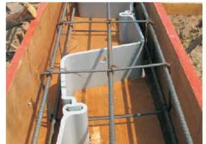
Tidewall was installed as a flood wall surrounding a valuable commercial installation. Thailand experienced a major flood in 2011, resulting in a need for cost-effective floodwalls throughout populated areas. Tidewall was an ideal solution; a 2 meter high wall finished with a steel reinforced concrete cap.
