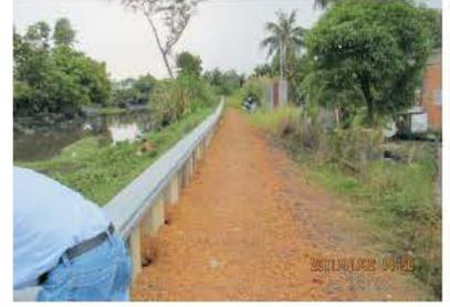
Tidewall was installed as a flood wall on several canals prone to flooding. The earthen dikes would erode and fail, allowing the flood waters to breach the dike. The Tidewall sheets were driven into the center of the dikes, with the wall projecting above the top of the dike to a specified height, providing a permanent solution to the flooding problems.
